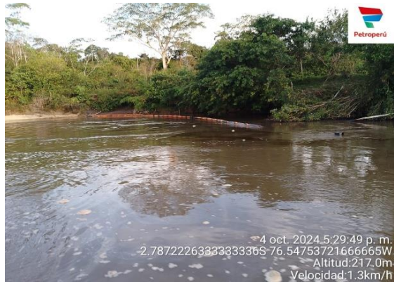
Picture 2. Installation of containment barriers on the Pastaza River (October 04, 2024).
