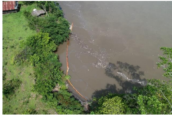
Picture 4. Installation of containment barriers on the Pastaza River. (October 04, 2024).
